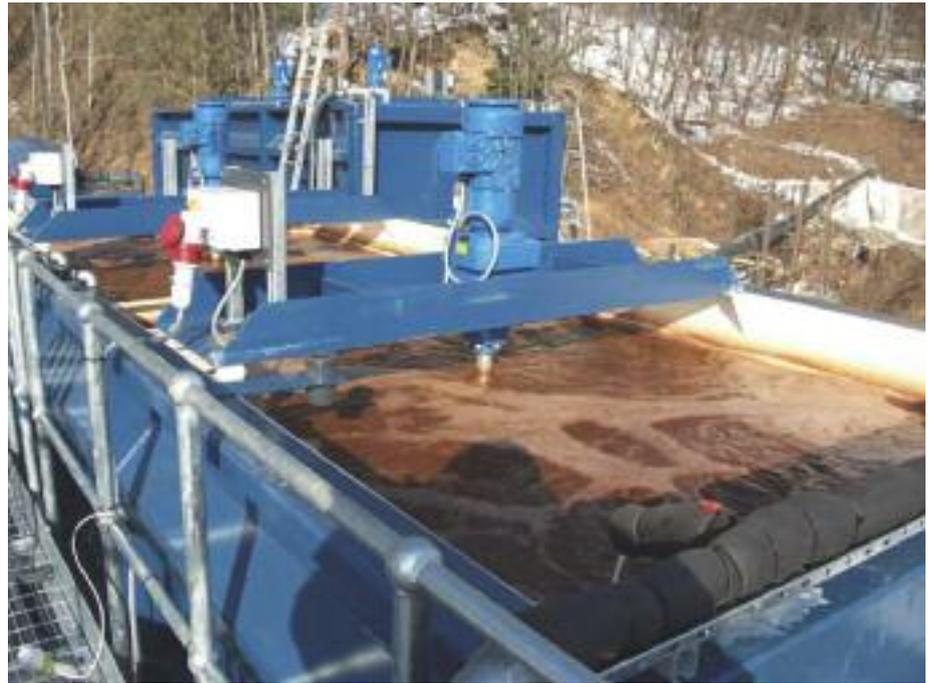
65 filter media. The captured iron is released during the filter backwash cycle.
